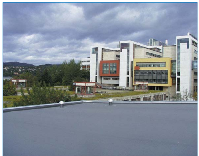
Vacuum vents in the corner zone
